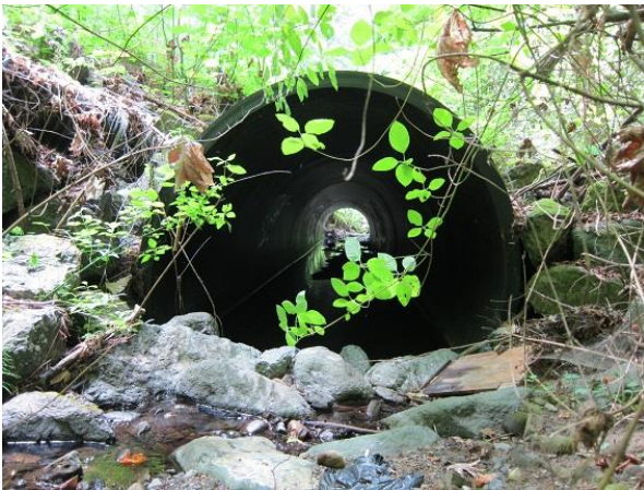
Culvert Inlet
