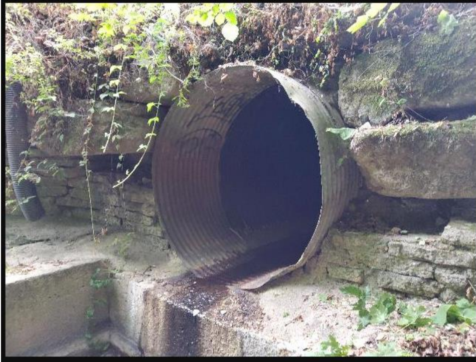
Outlet: Casserly Creek at Gaffey Road PM 0.80; Inside culvert, showing poor condition.
