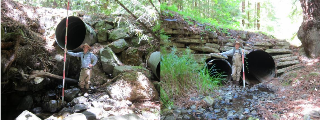
Left: Culvert Outlet; Right: Culvert Inlet
