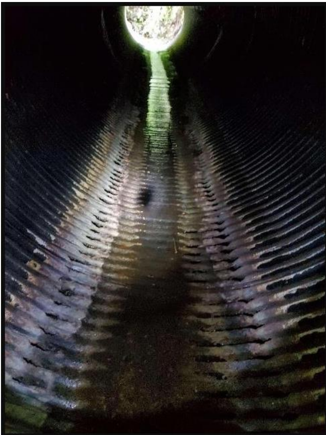
Outlet: Casserly Creek at Gaffey Road PM 0.80; Inside culvert, showing poor condition.
