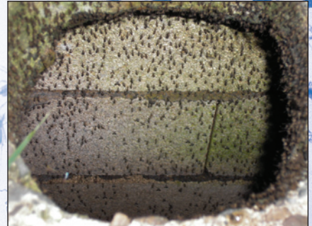
Mosquitoes in septic tank
